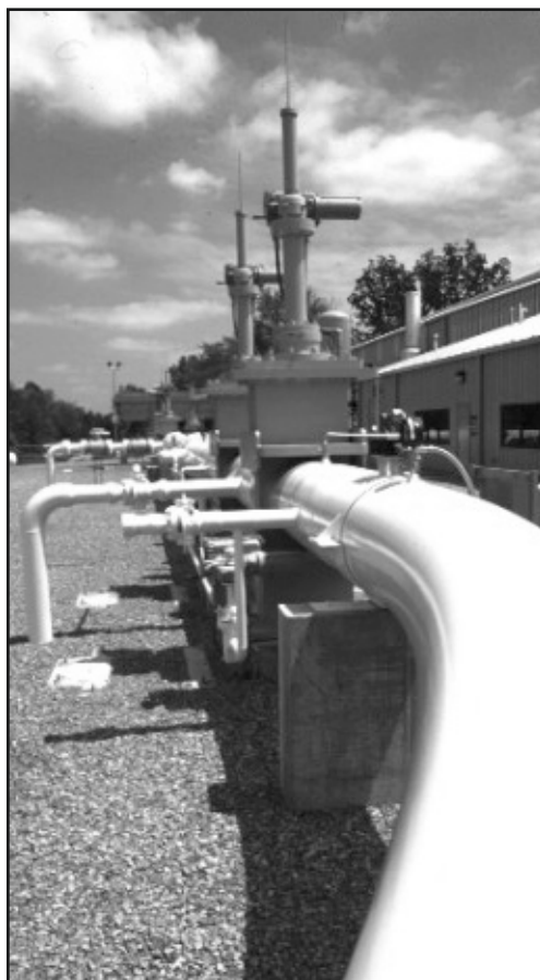
Photos courtesy of the Gas Technology Institute
